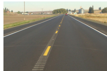
Install Centerline Rumble Strips
