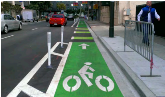
Install Separated Bicycle Lanes
