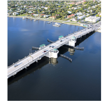
Southern Blvd. Bridge
