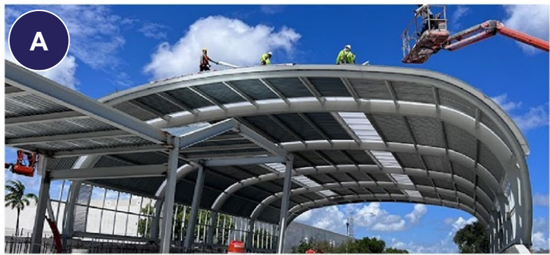
South Corridor: Bus Transit, under construction**
