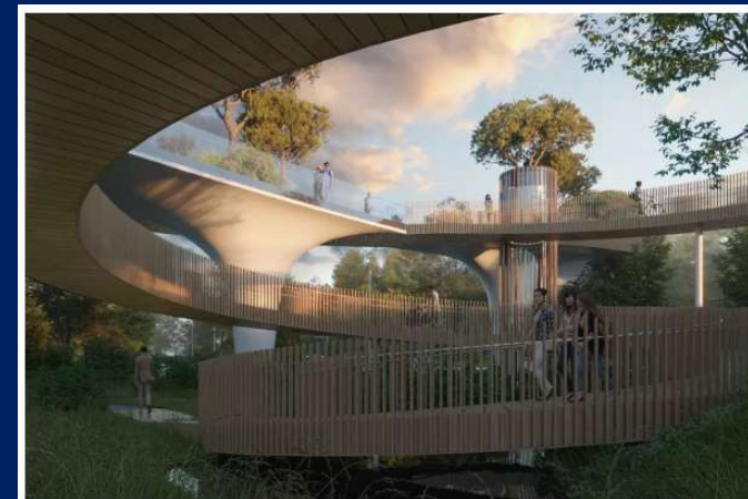
A spiral ramp up with a 5-degree incline takes pedestrians to the bridge.
