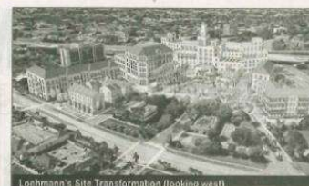
Loehmann's Site Transformation (looking west)
