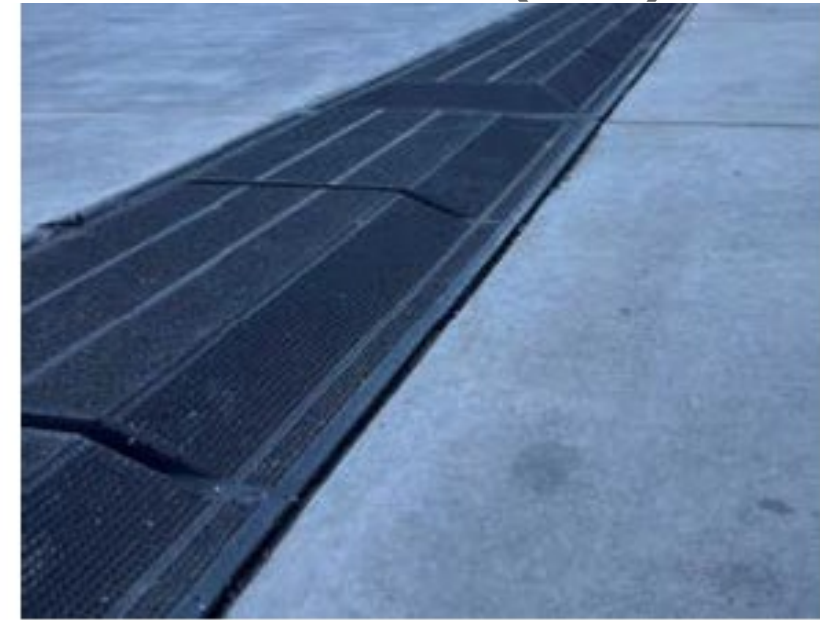
Tactile Warning Delineators (TWD)
