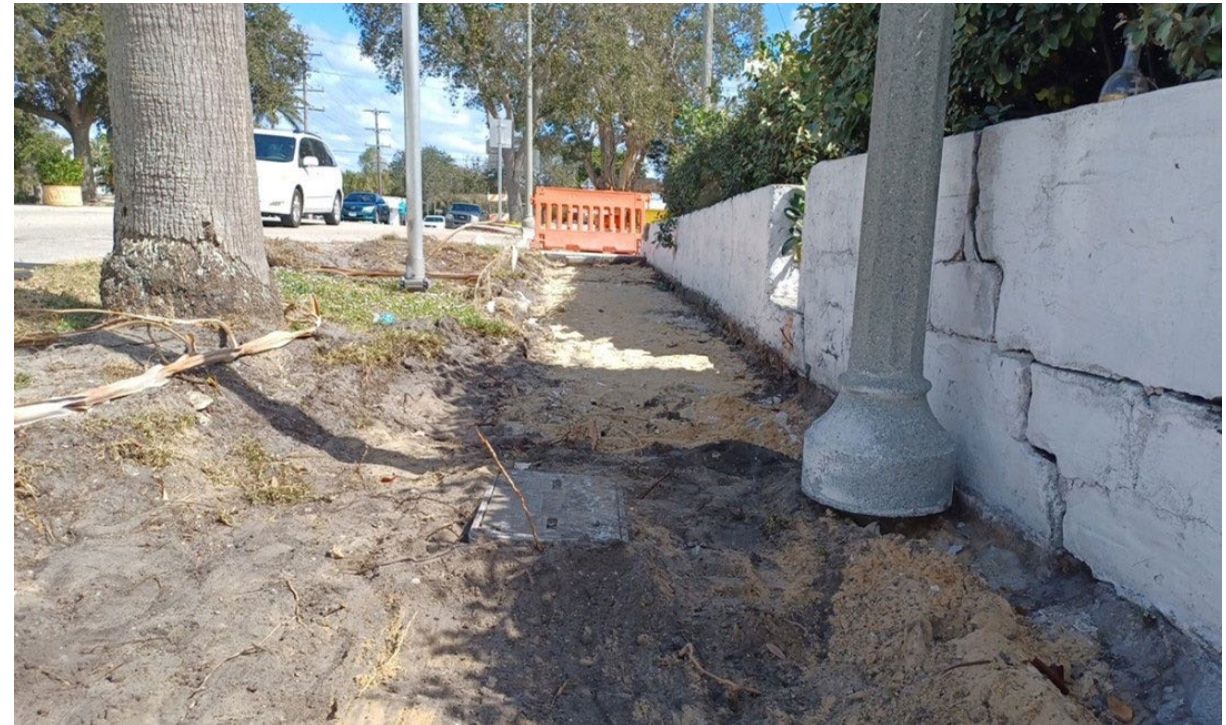
SR 802/Lake Worth Road Roundabout & Pedestrian enhancements – February 2024
