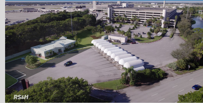
New Revenue Control Building
