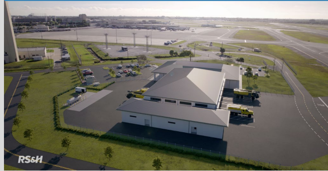
New Aircraft Rescue and Fire-Fighting (ARFF) Facility
