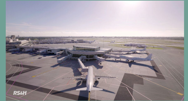
Concourse B Expansion
