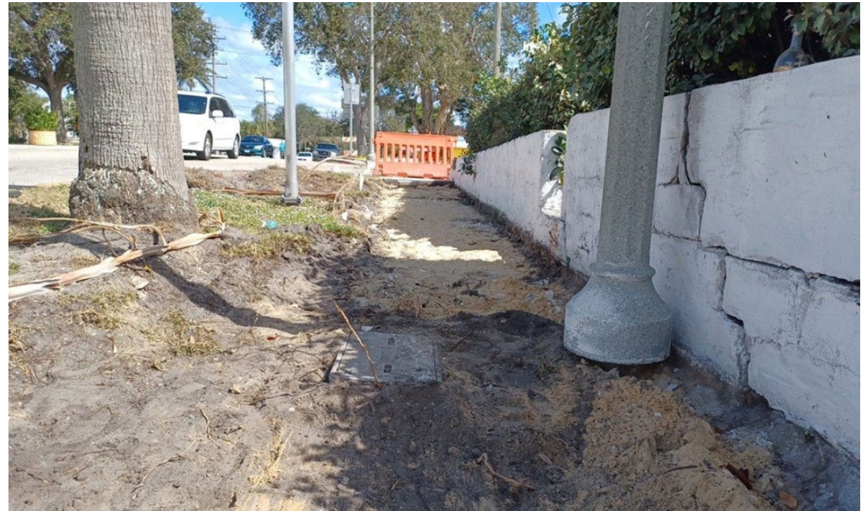
SR 802/Lake Worth Road Roundabout & Pedestrian enhancements – February 2024
