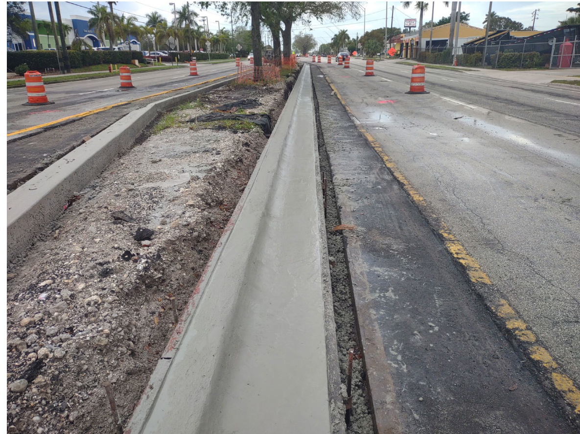
Lake Worth Rd Reconstruction – new curb & gutter March 2024
