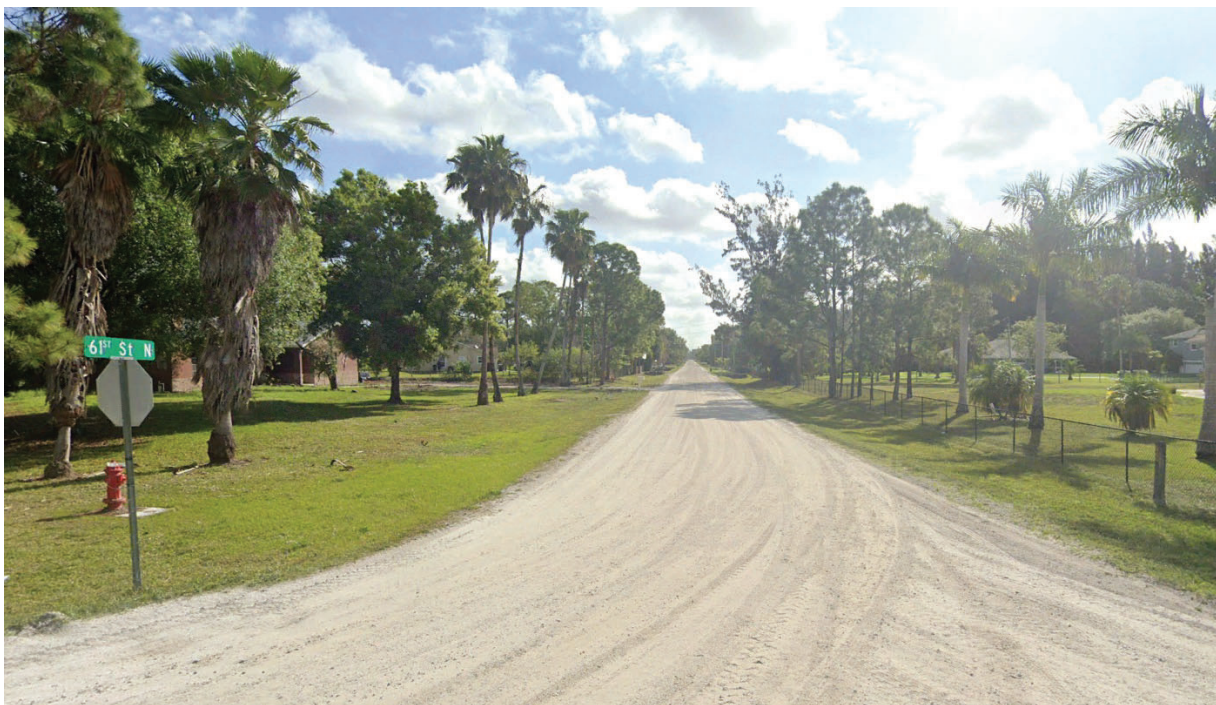
#2 - 61st St N & 140th Street North Facing East
