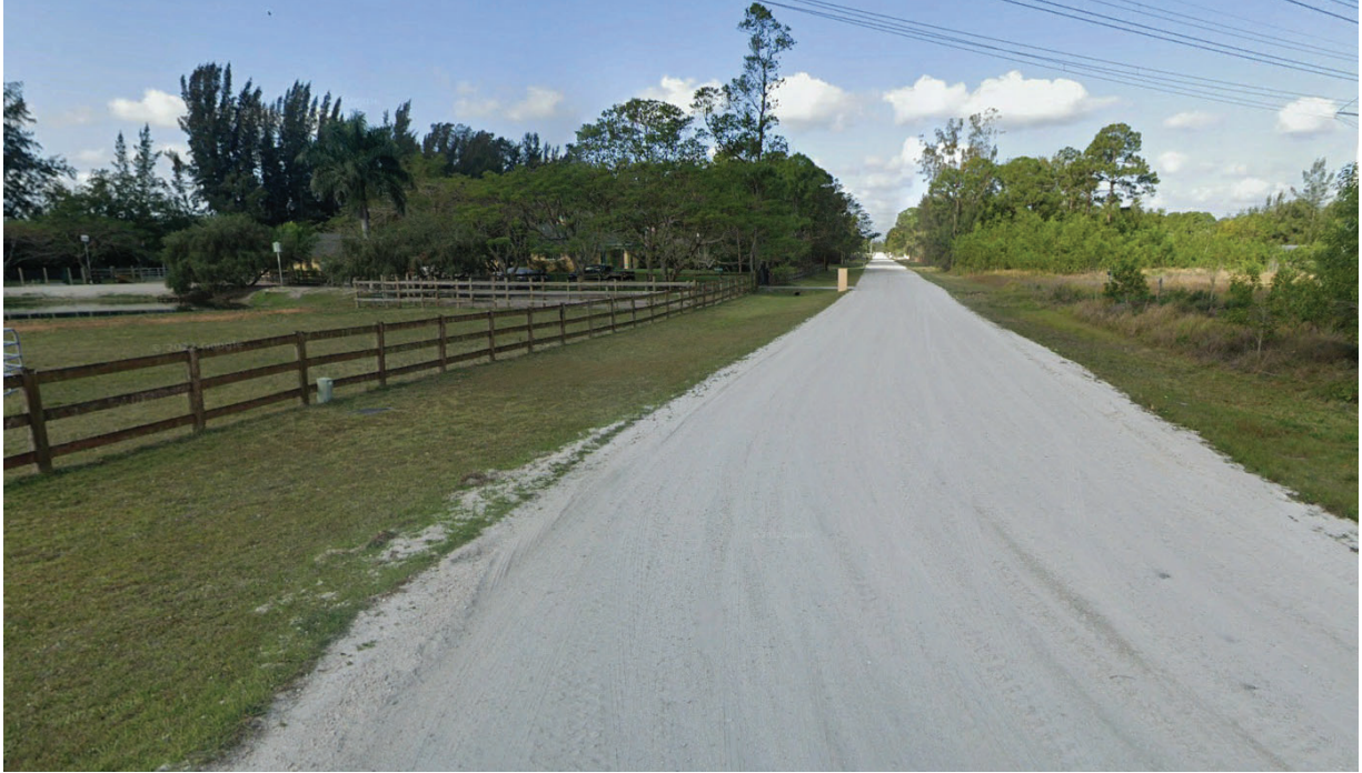
#2 - 61st Street N & M-1 Canal Facing West
