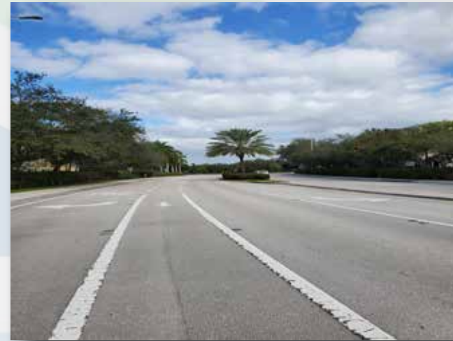
South Approach - Looking North
