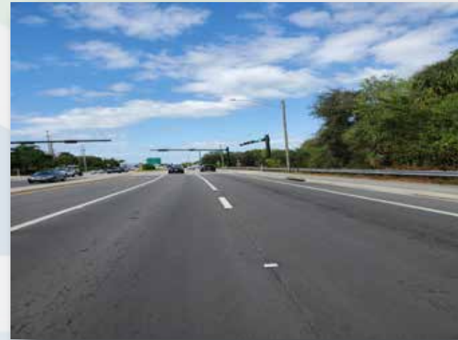
East Approach - Looking West
