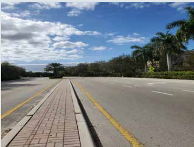
South Approach - Looking South
