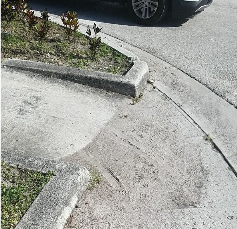
Evidence of erosion, and lacking ADA along Military Trail; Photo by: CTS Engineering, Inc.
