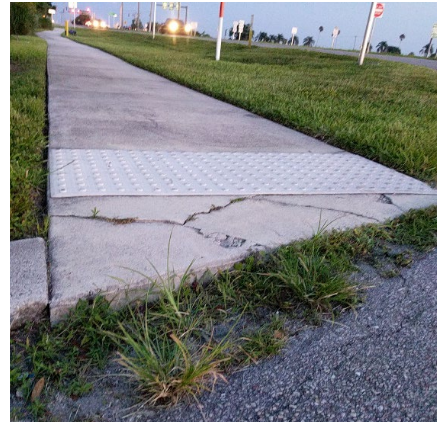
Sidewalk drops off at service center, possible hazard; Photo by: CTS Engineering, Inc.
