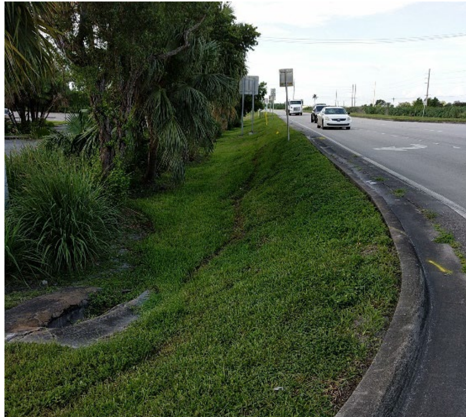
No sidewalk or handrail on N. Main St., south of Hooker Highway; Photo by: CTS Engineering, Inc.
