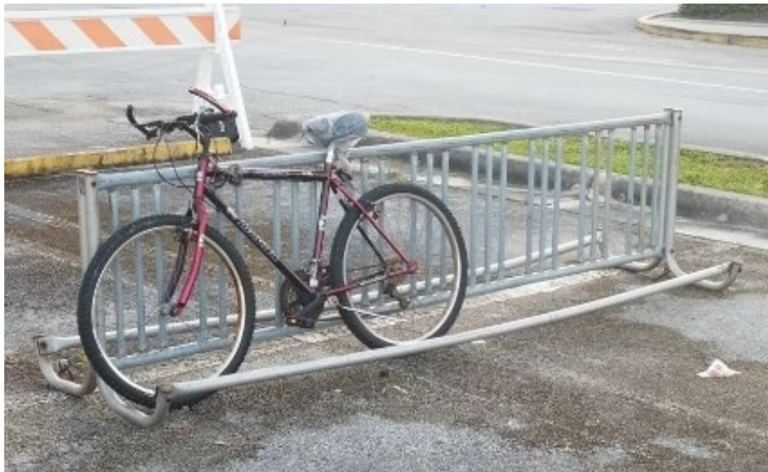
Bicycle rack at mall bus stop (687); Photo by: CTS Engineering, Inc.
