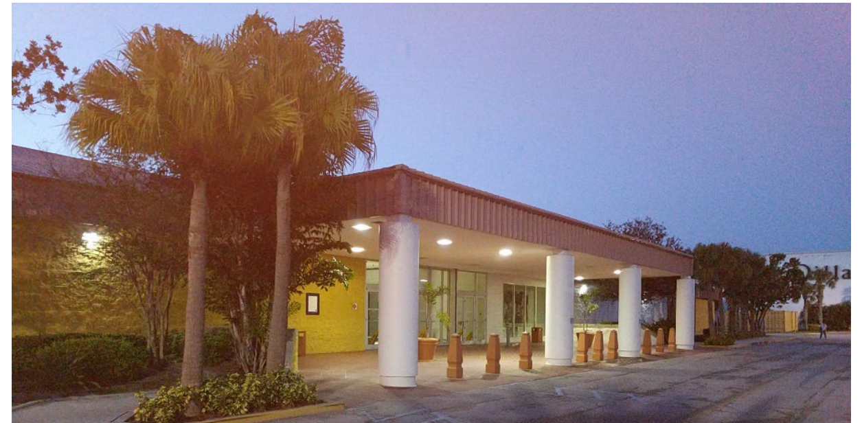
Building offering light at stop at mall; Photo by: CTS Engineering, Inc.
