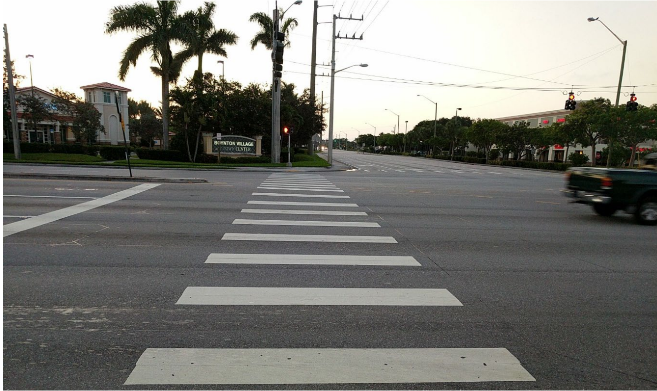
Crosswalk at intersection of Old Boynton and Congress; Photo by: CTS Engineering, Inc.
