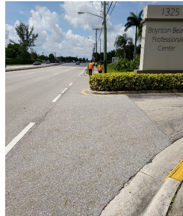
Median needs pulled back at Professional Center on S. Congress; Photo by: CTS Engineering, Inc.
