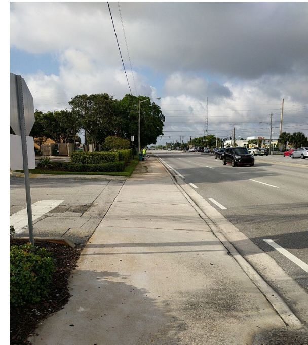
8 ft sidewalks near N. Congress and Boynton Beach Boulevard intersection; Photo by: CTS Engineering, Inc.
