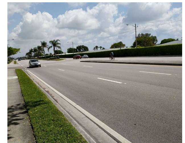
Road conditions along corridor; Photo by: CTS Engineering, Inc.
