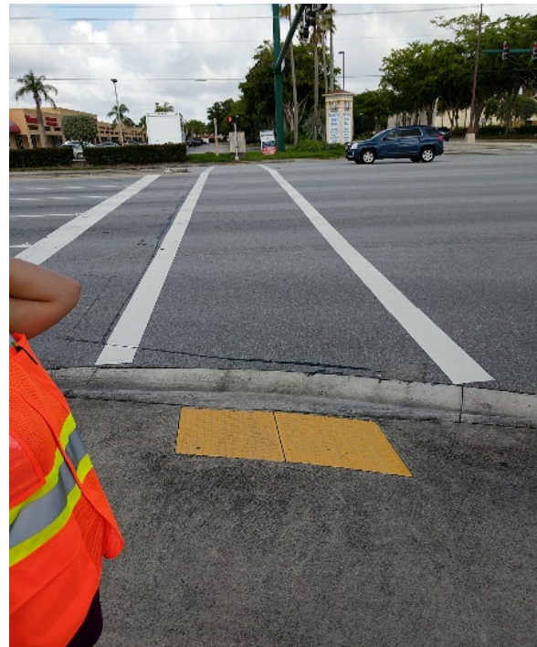
Crosswalk needed at Congress & Boynton Town Center; Photo by: CTS Engineering, Inc.
