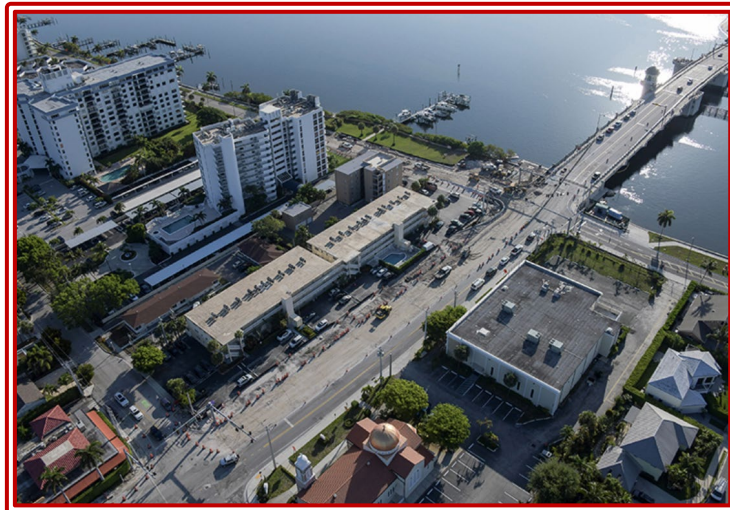
Continuous progress being made on the Bridge Replacement. May 2023
