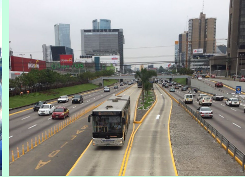
Center Platform Bus Rapid Transit
