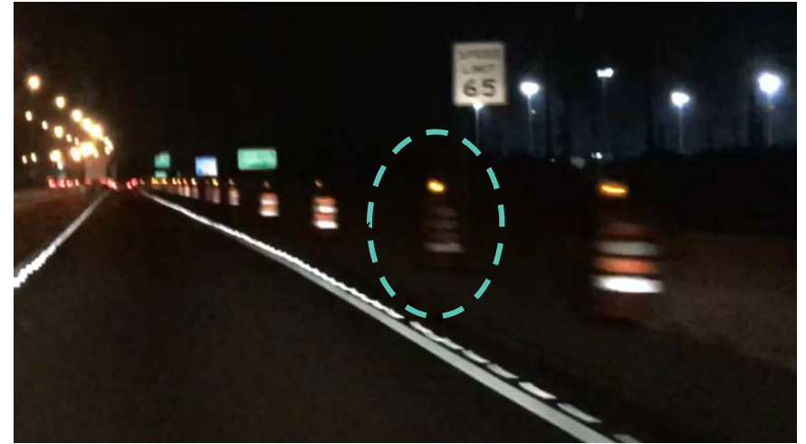
Figure 10: Non Reflective Barrel
