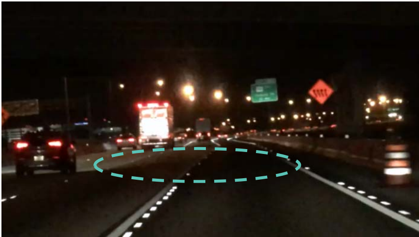
Figure 9: RPMs in Tangent Section
