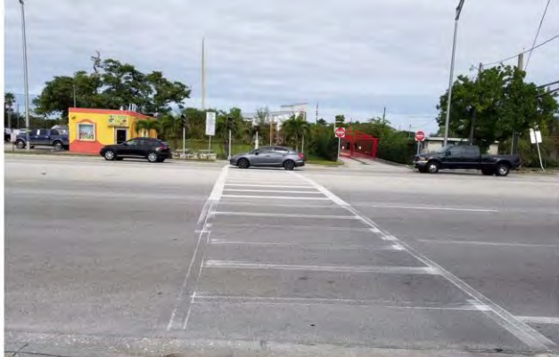
Faded crosswalk markings at Emergency Signal/Swap Shop. Looking north.
