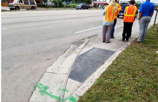
Substandard detectable warning surface at Price Street. Looking west.
