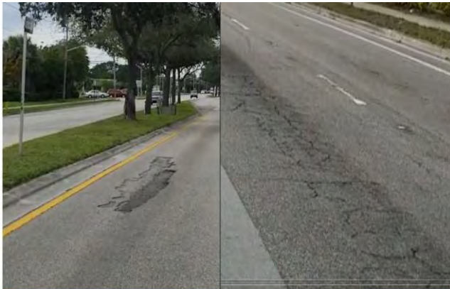
Potholes and cracking in the pavement. Eastbound lanes.
