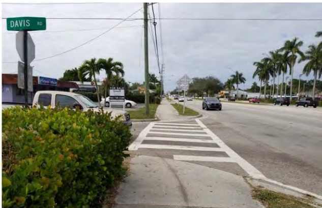
No detectable warning surface provided at Davis Road. Looking west.
