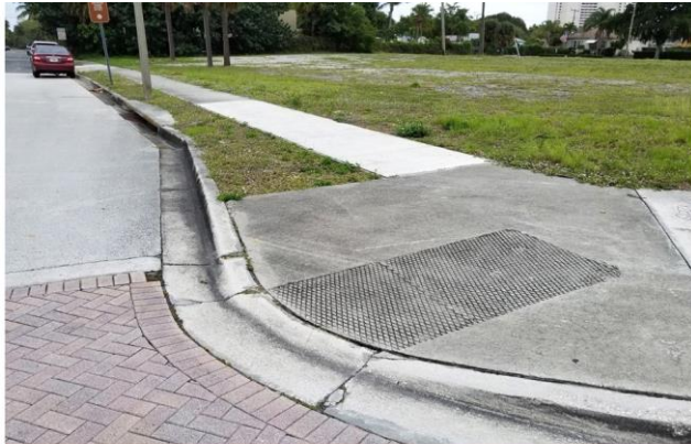
Typical curb ramp with substandard detectable warning surface along corridor.
