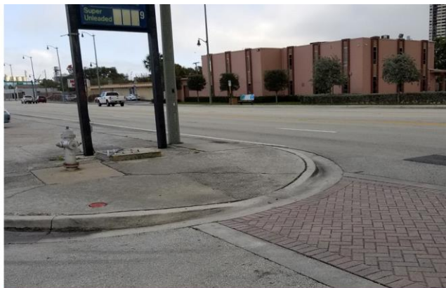
Substandard detectable warning surface at 52 nd Street. Looking north.
