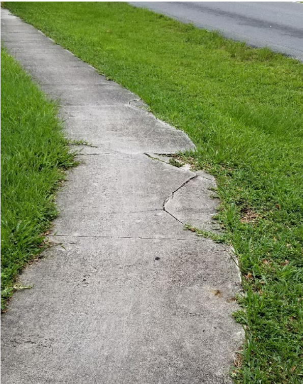
Narrow, broken sidewalk along corridor; Phot by: CTS Engineering, Inc.
