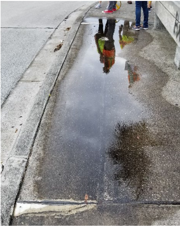
Puddling water on sidewalk along corridor; Photo by: CTS Engineering, Inc.
